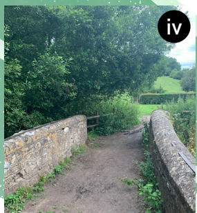
iv Cross the Siston Brook using this bridge. The brook is a tributary for the River Avon and was once used to provide power for watermills and battery mills.
